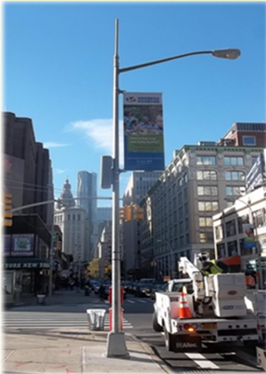
(AT&T node on municipal light pole in Manhattan)
