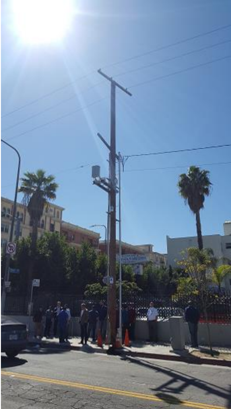
(AT&T installation on existing utility pole in Los Angeles with electric distribution and other telecommunication installations)
