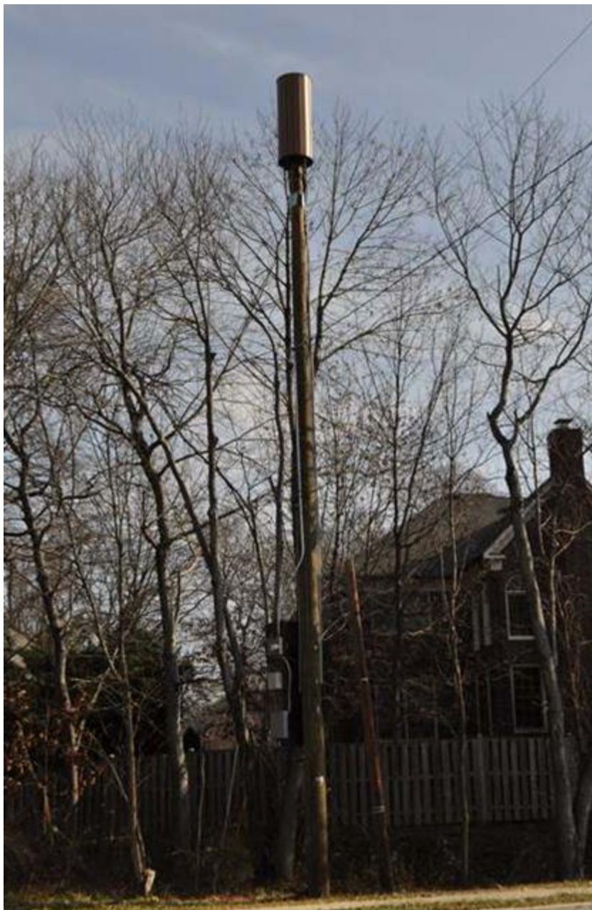
(AT&T installation in Hunter Mill, VA)
