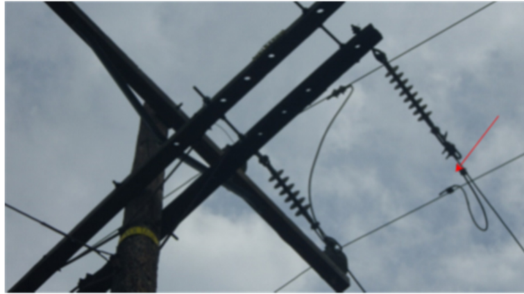
Figure IV-21 Visual Inspection View
