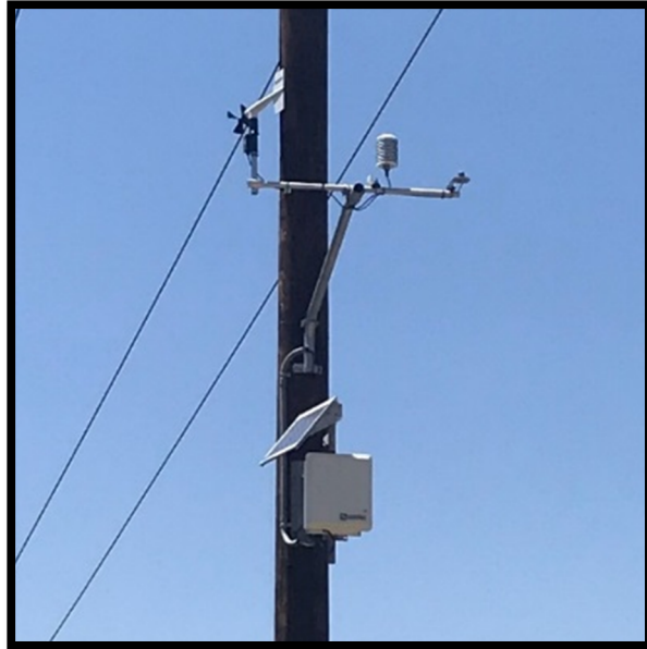
Figure IV-19 SCE Weather Station on Distribution Pole
