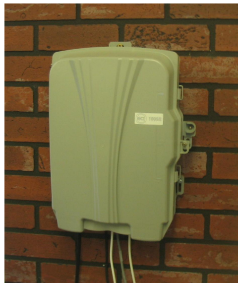
Example – External Mounted ONU
