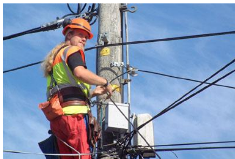
Example – Aerial Feeder Cable Installation
