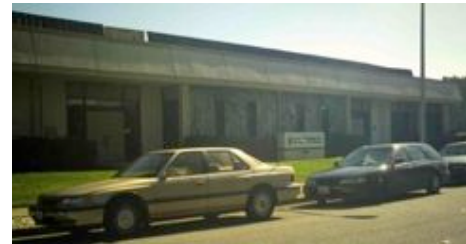
Figure 5.11 - Typical building and company on East Meadow Circle.
